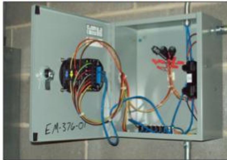
This meter, installed at a facility on Redstone Arsenal in 2009, provides customers with a centralized view of energy and water consumption, energy efficiency and energy management.
