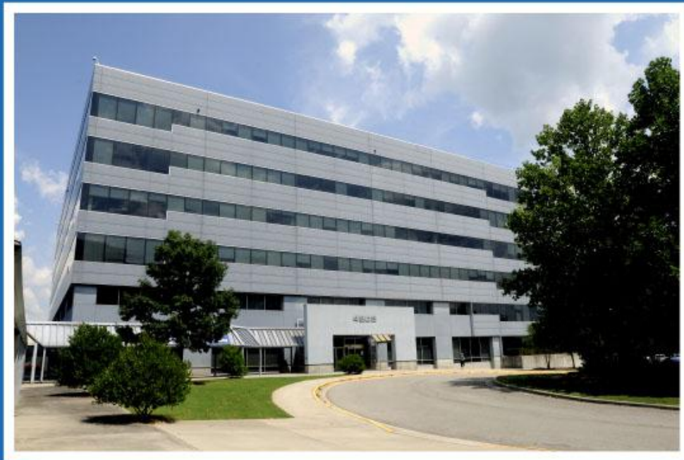
Building 4203 Constructed 1992 Registered as LEED EBOM 2008 (Existing Building Operations and Maintenance) Marshall Space Flight Center Huntsville, Alabama
