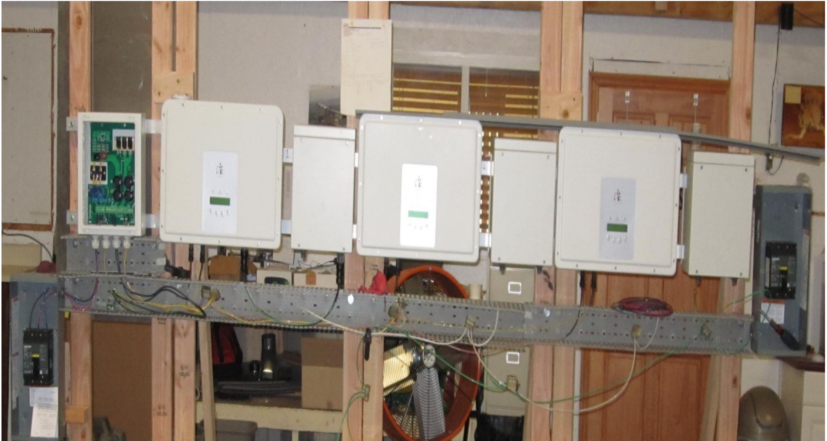
480/277-Y 3-Phase Grid Tie
