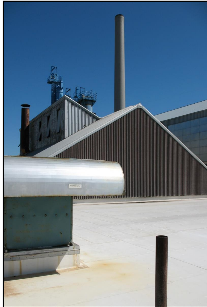
AFTER GEM Steam Trap retrofit
