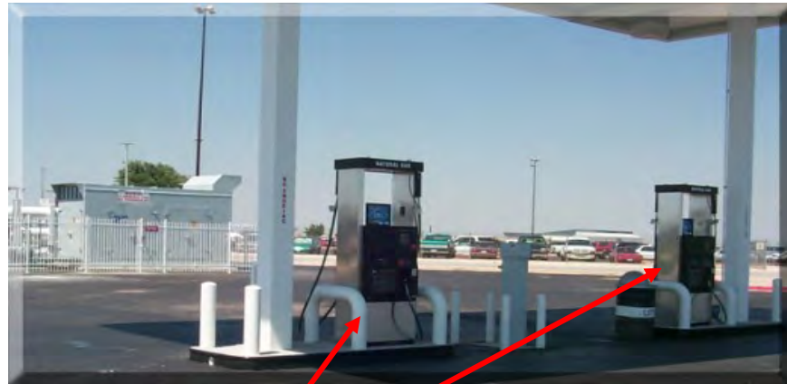
Two hose fueling dispensers with internal sequencing
